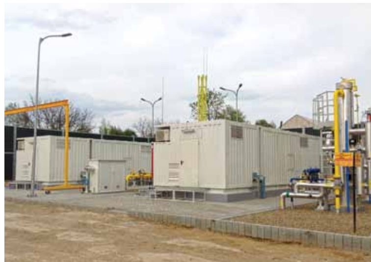
■ EGS made these 420 hp (315 kW), 1000 rpm ABB electric-motor-driven Ariel JGE/2 single- and two-stage compressor packages for Polish EPC contractor PGNiG Technologie. The systems are inside explosion-proof, noise-suppressing enclosures.
