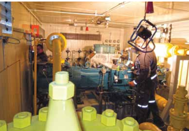
■ EGS made these 420 hp (315 kW), 1000 rpm ABB electric-motor-driven Ariel JGE/2 single- and two-stage compressor packages for Polish EPC contractor PGNiG Technologie. The systems are inside explosion-proof, noise-suppressing enclosures.
